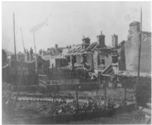
Bomb damage to cottages at East Cowes
